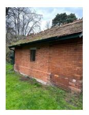
Pavilion pointing to brickwork where extension was removed needs attention. Specialist required to blend brick colours to match. Rubbish to be cleaned off roof. Any proposal to install security gates should be done in consultation with Howley Hayes Conservation Architects.
